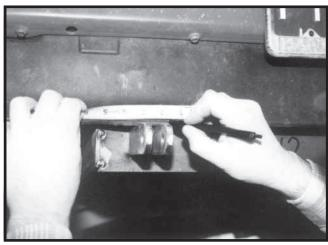
Mark the 1-5/8" x 2-1/2" slots by using the pulling ears of the base plate to guide you in the loacation.
